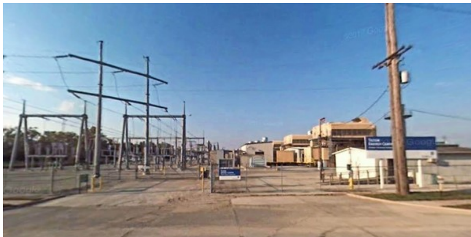
Tilton Energy Center | Google
