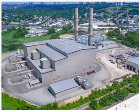
North Bergen Liberty Generating Plant | Diamond Generating
