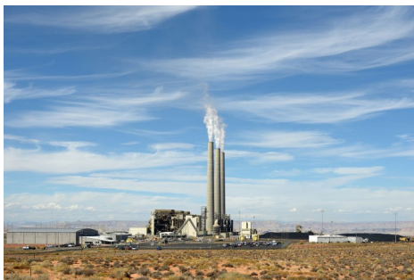
Navajo Generating Station
