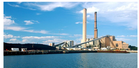
Salem Harbor Power Station | Tetra Tech
